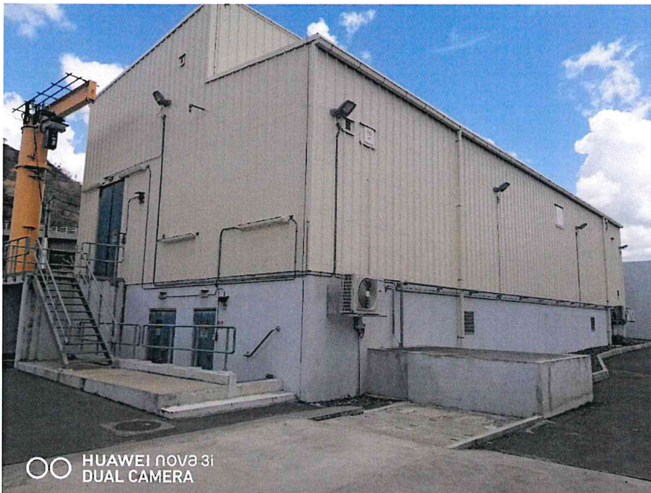
(Existing GIS sub-station at the Saint Louis Power Station, Mauritius)
